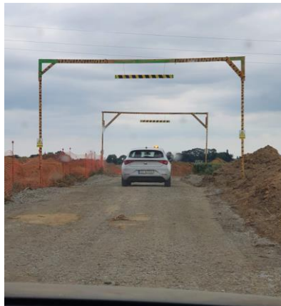
Photo So called gantry cranes in front of high-voltage lines
